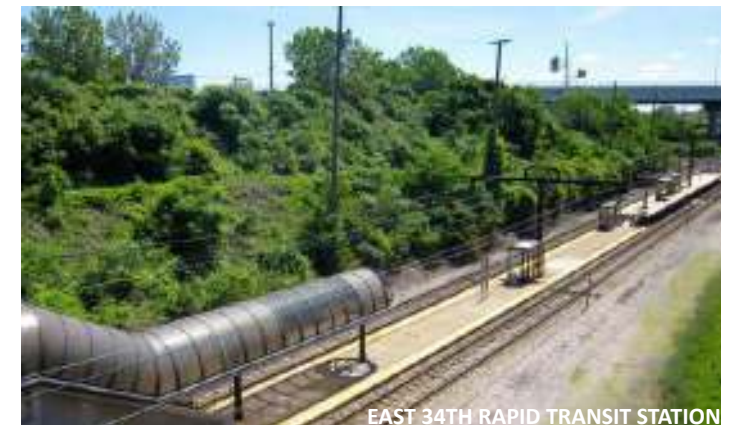
EAST 34TH RAPID TRANSIT STATION
